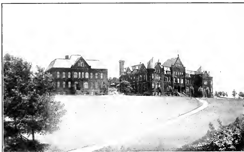
The Present Buildings of the University Science Hall The Main Building
