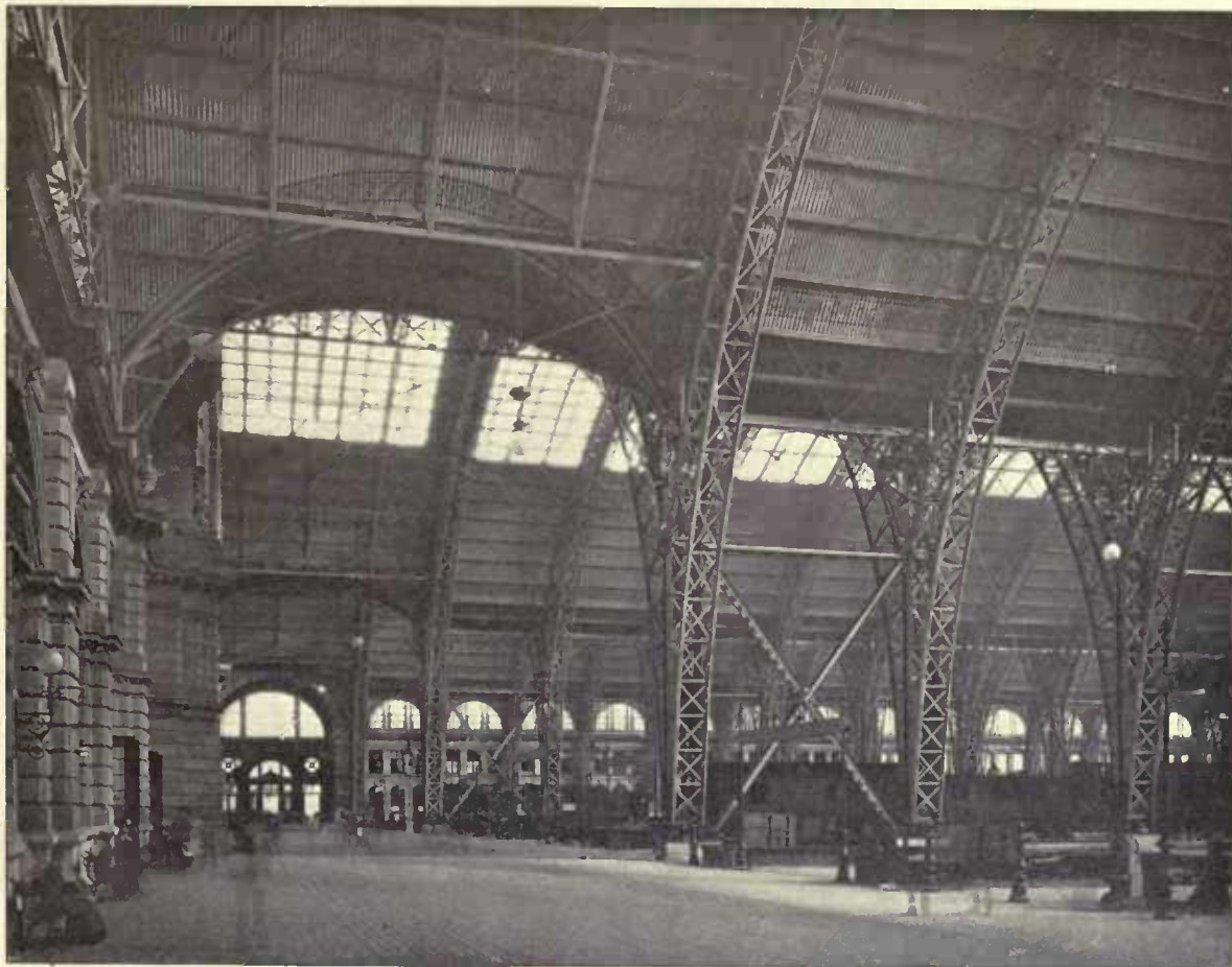
INTERIOR OF THE TRAIN SHEDS OF THE FRANKFORT RAILWAY STATION; ENTIRELY OF METAL AND GLASS
