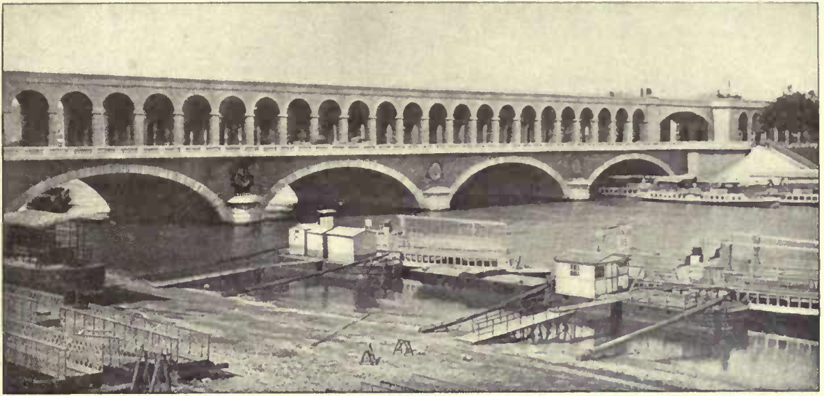
THE AUTEUIL VIADUCT, PARIS ELEVATED RAILROAD IN CENTRE OF DRIVEWAY
