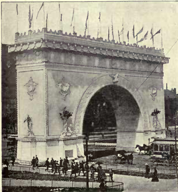
CENTENNIAL ARCH, CLEVELAND, O.
