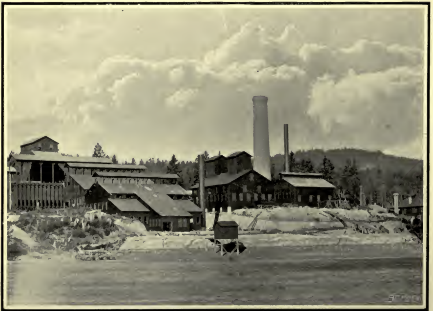
NORTHWESTERN SMELTING & REFINING CO., CROFTON, V. I. B. C.
