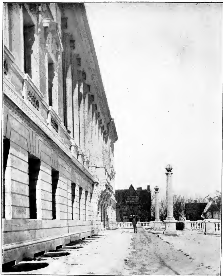
East façade of State Historical Library, in Winter
