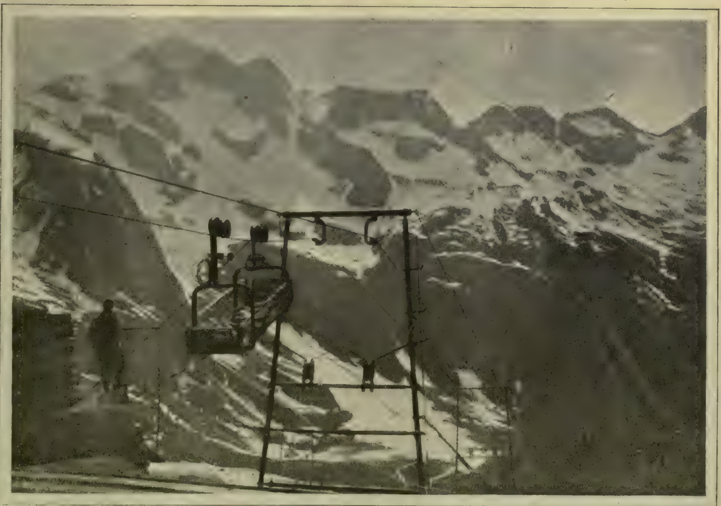
Preparing to Start
