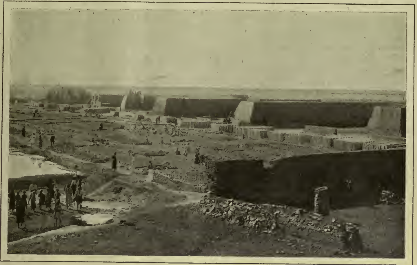
The New Hindia Dam
