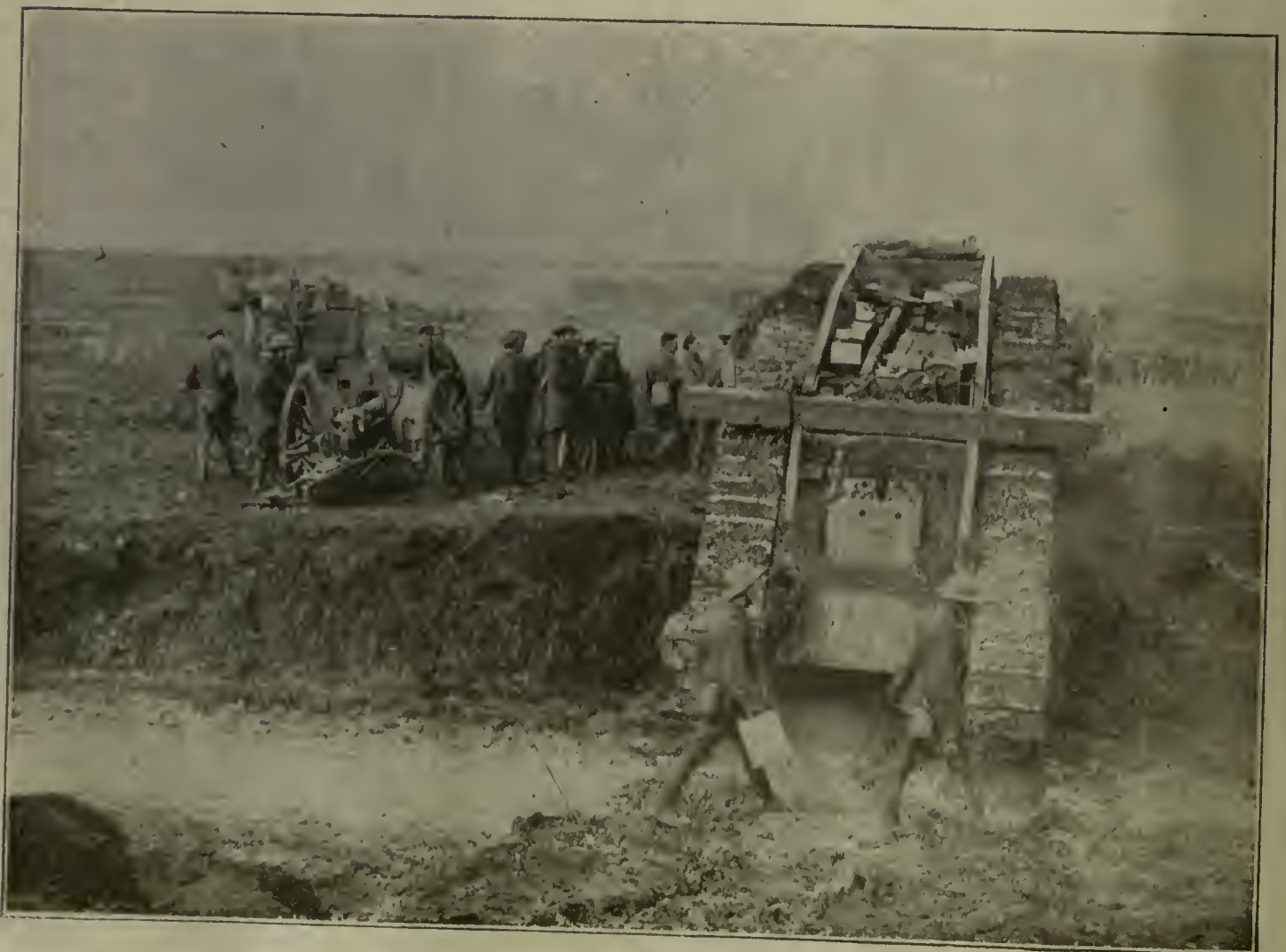
Tanks on the way to Bournon Wood
