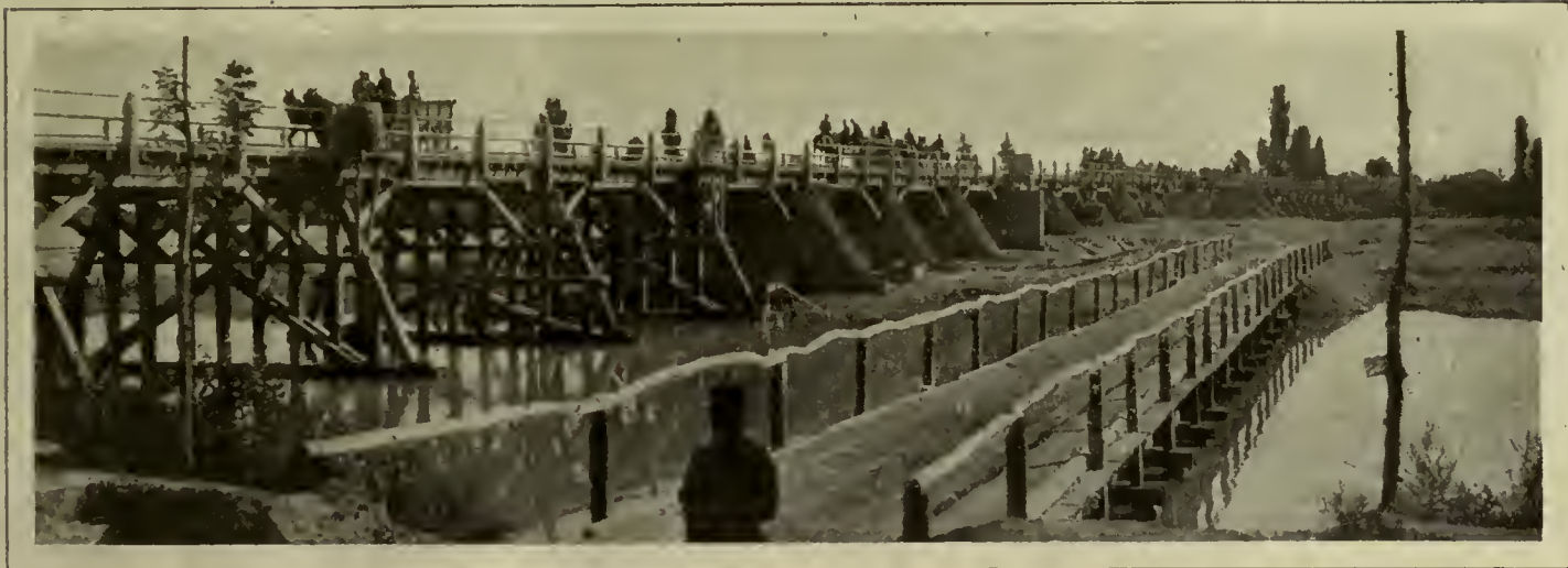
Bridge over the Tagliamento
