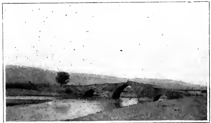
Bridge over Canal
