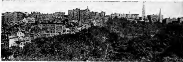
VIEW FROM THE SCHOOL OVERLOOKING THE PUBLIC GARDEN AND BEACON ST.
