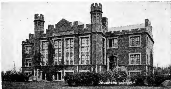
MAIN ACADEMY BUILDING
