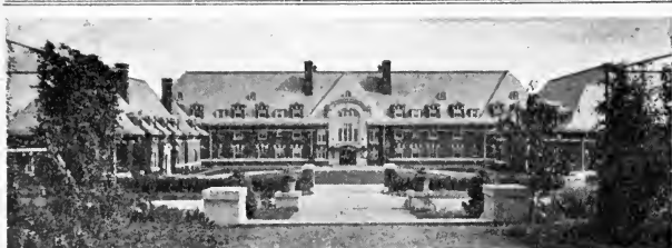
VIEW OF THE BUILDING FROM THE WEST. THE H SHAPE FORMS TWO COURTS, EAST AND WEST
