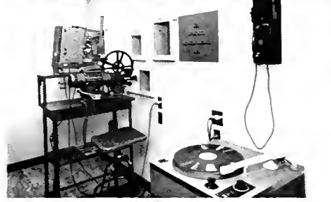
(Three views at right, top of bottom) dual 16mm projectors and turntables serve both assembly room areas. (Center) Projection booth showing dual level construction. Lower level for editing, shipping, etc.; upper level for projection and sound distribution to preview and assembly rooms. (Bottom) Preview room projection facilities shown in this view.
