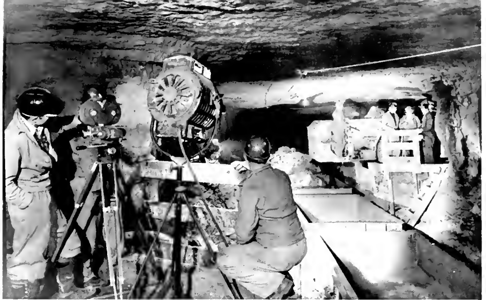
PREPARING TO SHOOT A TYPICAL SEQUENCE for one of the Joy Manufacturing Company color motion pictures at the Annandale, Pennsylvania limestone mine.
