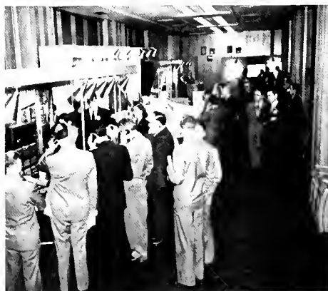
COMBINED ASSEMBLY ROOMS are shown in use for exhibit area of Bell System progress.
