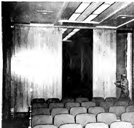
SOUNDPROOF FOLDING DOORS which create two rooms are easily handled by one man.
