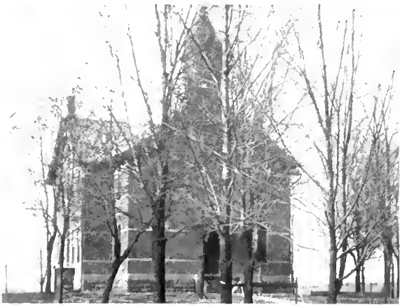
PUBLIC SCHOOL BUILDING, SUNBURY
