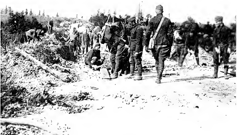
"Fighting through a tangled wilderness of shattered woods." ENGINEERS REPAIRING ROADS IN ARGONNE.
