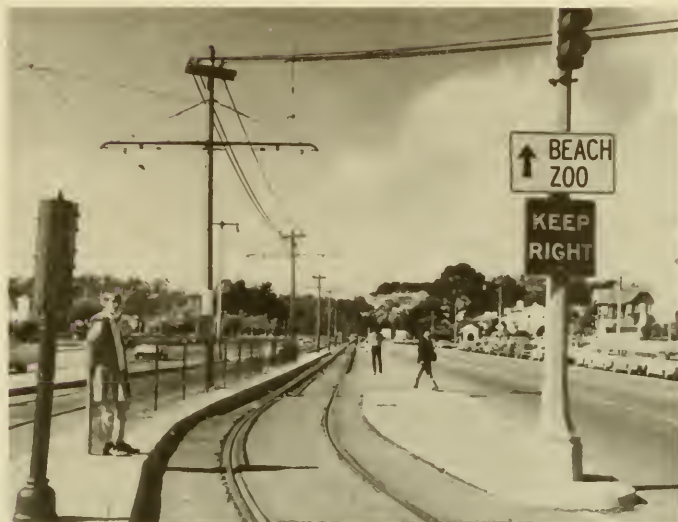
BEFORE-Overhead feeder cables and streetcar trolley overhead
