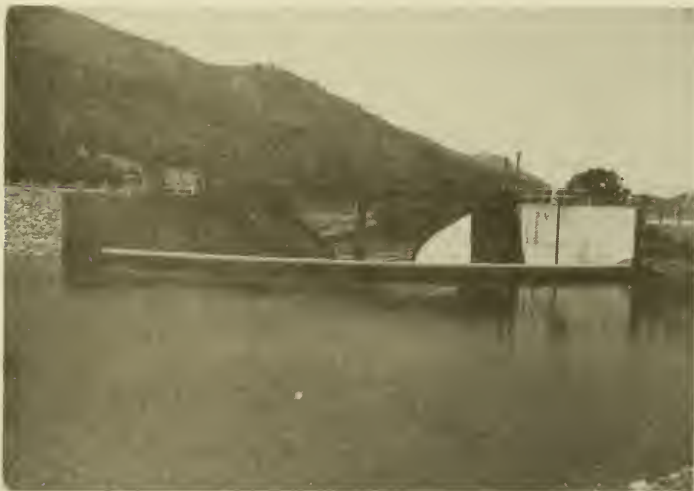
The completed Moccasin Spillway at the approximate site of the Diversion Flume Reconstruction completed March 18, 1976.
