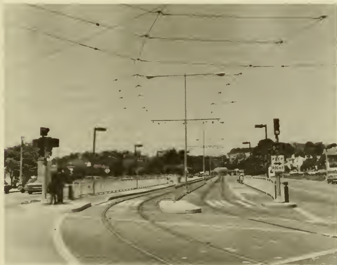
AFTER-New trolley/streetlight poles and pantograph type overhead
