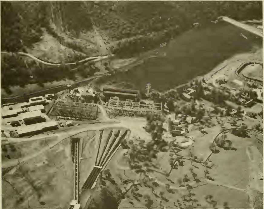
MOCCASIN POWERHOUSE AND RESERVOIR
