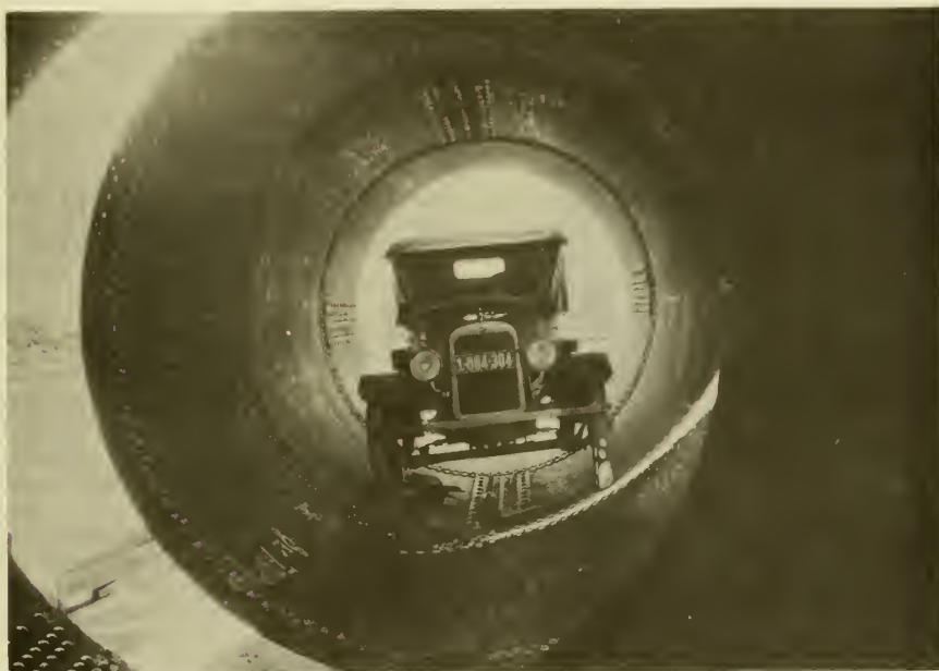
PHOTO TAKEN DURING CONSTRUCTION OF HETCH HETCHY AQUEDUCT, 9'6" PIPE, MARCH 1925
