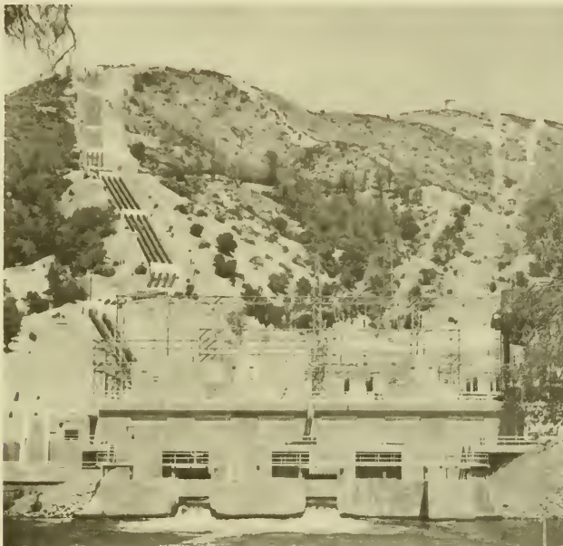
NEW MOCCASIN POWERHOUSE AND PENSTOCK
