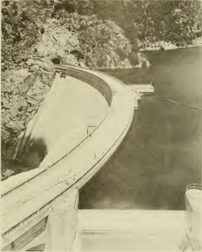
O'Shaughnessy Dam as it looks now.
