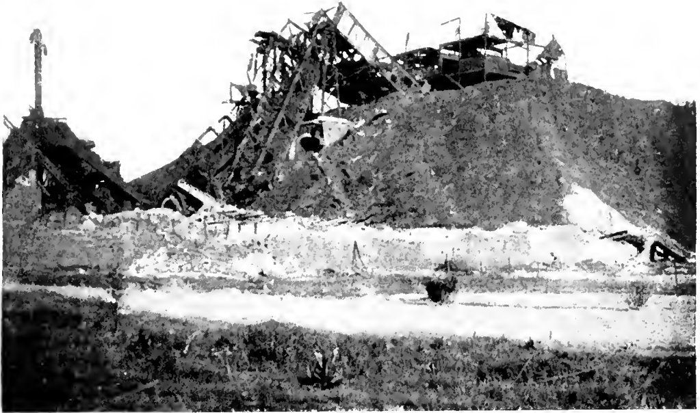
LOOS CRASSIER, WITH BROKEN PYLONS.
