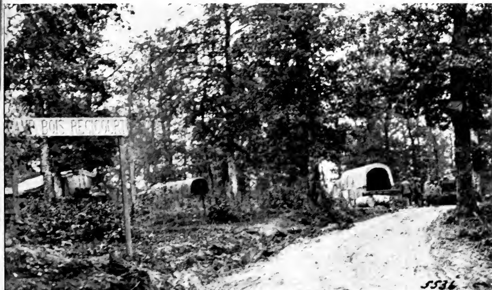
NEAR P. C. SEVIER, ENTRANCE TO REST-CAMP
