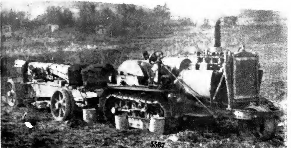
B AT GESNES, READY TO MOVE TO SEDAN
