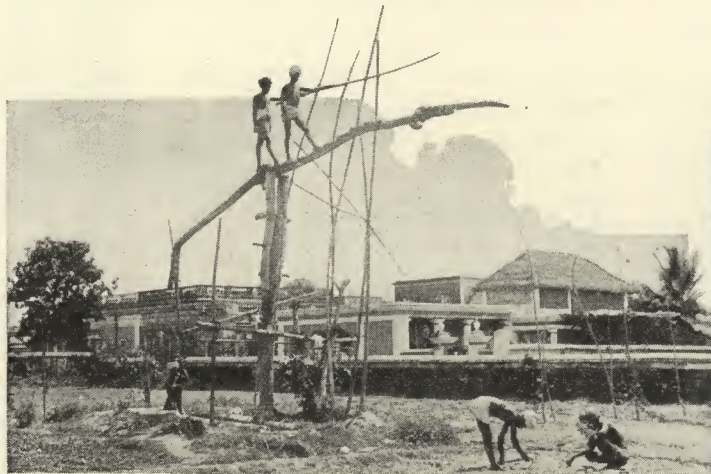
Far away, in India, natives "Walk the Plank" to raise water to the ground level.
