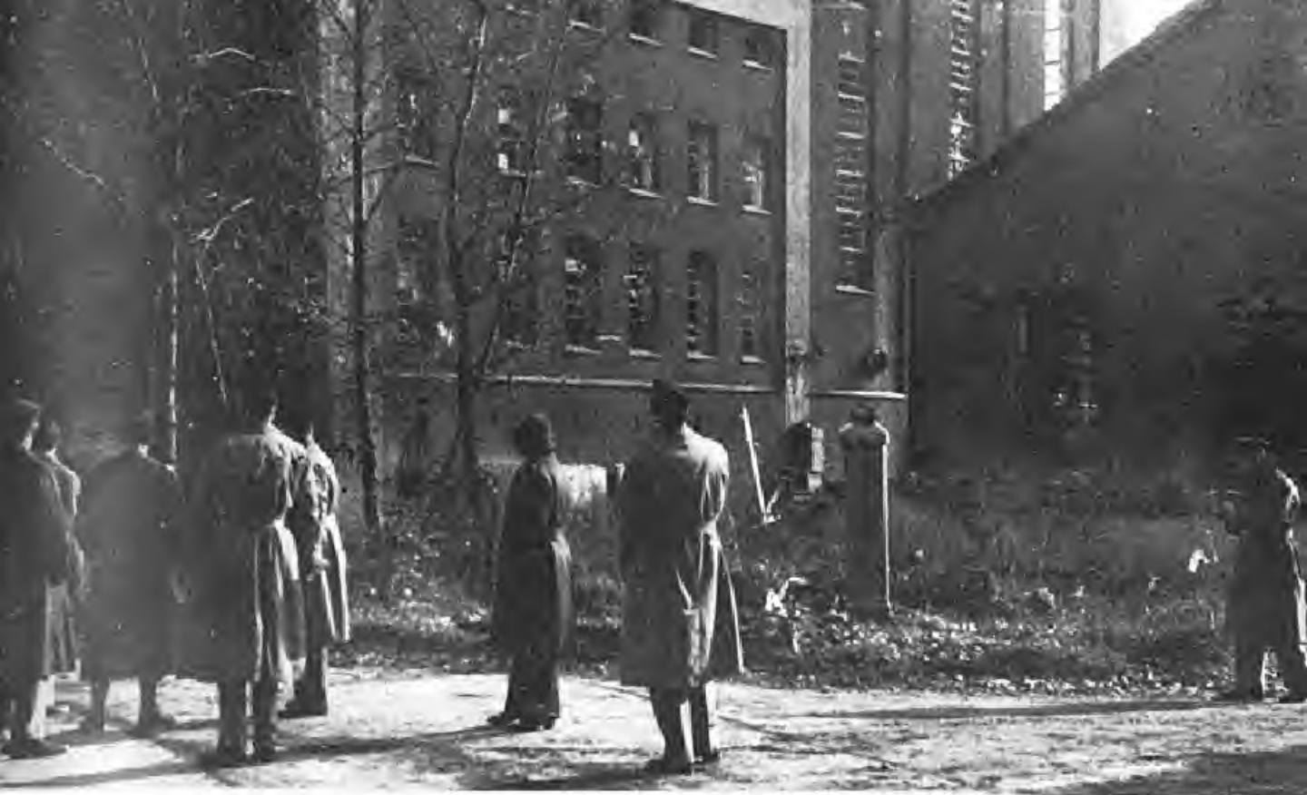
I. G. Farben military explosives plant at Ebenhausen, before and after demolition operation.
