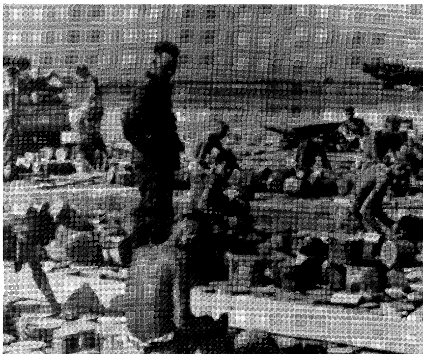
German airfield construction in Russia, 1941. Reich Labor Service battalions pour footings and emplace primitive but durable wood stump taxiways.
