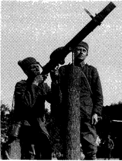
Improvised anti-aircraft machine gun emplacements. (Left) American troops use log as pedestal for Lewis gun. Gunner of the French 65th Anti-aircraft Autocannon Section aims skyward. (Below) German tub emplacement rotated to allow a 360 degree arc of fire. U.S. Army Air Defense Museum.
