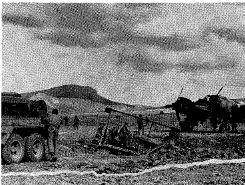
D-7 bulldozer fills crater torn into a North African airfield. Rapid repairs ensured near continuous operations.
