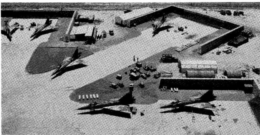
American F-102s shelter behind gravel filled prefabricated steel revetments at Da Nang, South Vietnam, July 1966.
