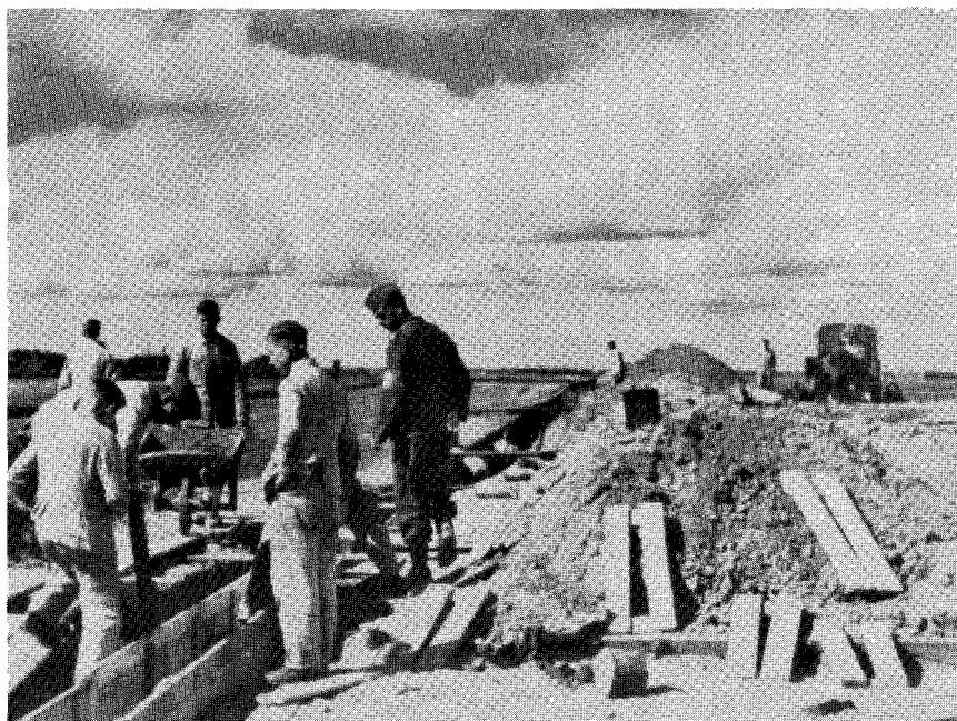
German airfield construction in Russia, 1941. Reich Labor Service battalions pour footings and emplace primitive but durable wood stump taxiways.
