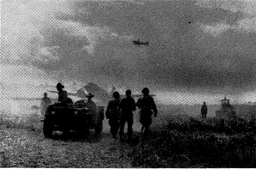
C-47s land at strip at Nadzab, New Guinea, while engineers are still laying out the facility. Mobility and surprise were the hallmarks of Kenney's operations.
