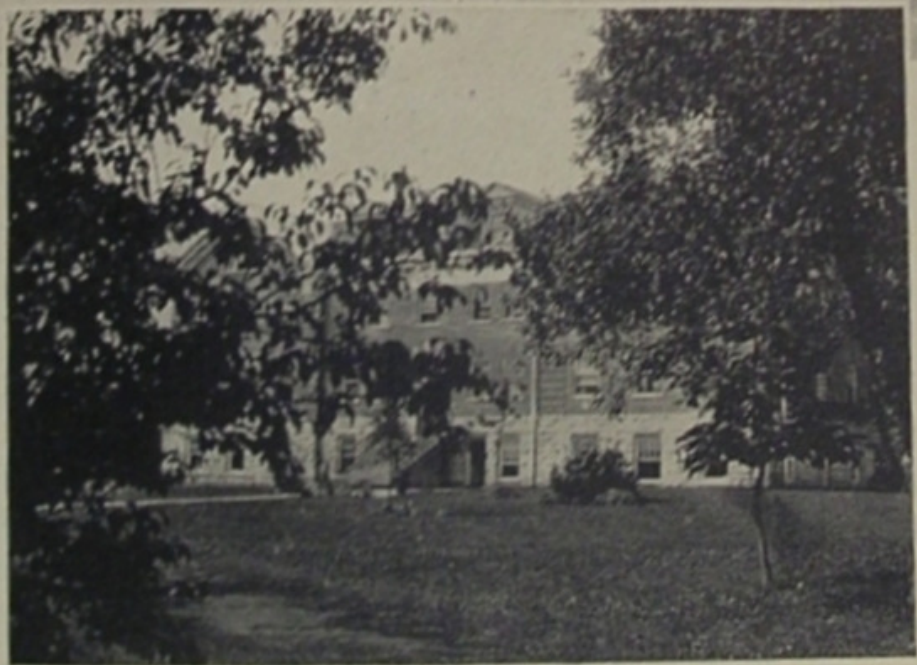
METCALF HALL STEAM PLANT AND LAUNDRY WEST HALL
