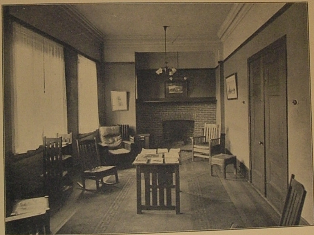
DOMESTIC SCIENCE HATHAWAY PARLOR
