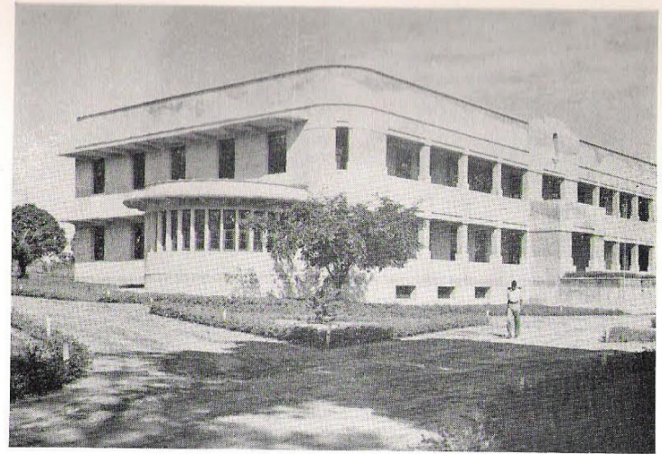
THE BELGIAN CONGO HAS BEEN DESCRIBED AS THE MOST MODERN OF AFRICAN COLONIES. BUILDINGS LIKE THIS CONTRIBUTE TO THAT IMPRESSION
