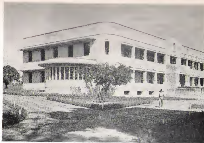
THE BELGIAN CONGO HAS BEEN DESCRIBED AS THE MOST MODERN OF AFRICAN COLONIES. BUILDINGS LIKE THIS CONTRIBUTE TO THAT IMPRESSION
