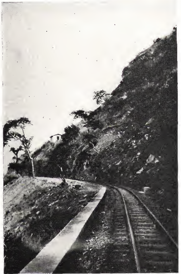
Many obstacles were overcome to build the railway
