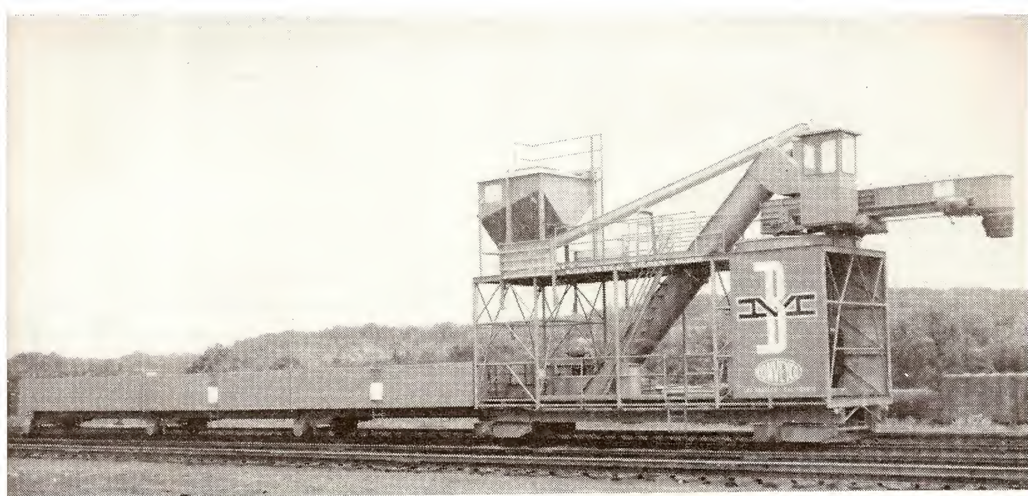
Boston and Maine's ultra-modern, rail mounted train icer.
