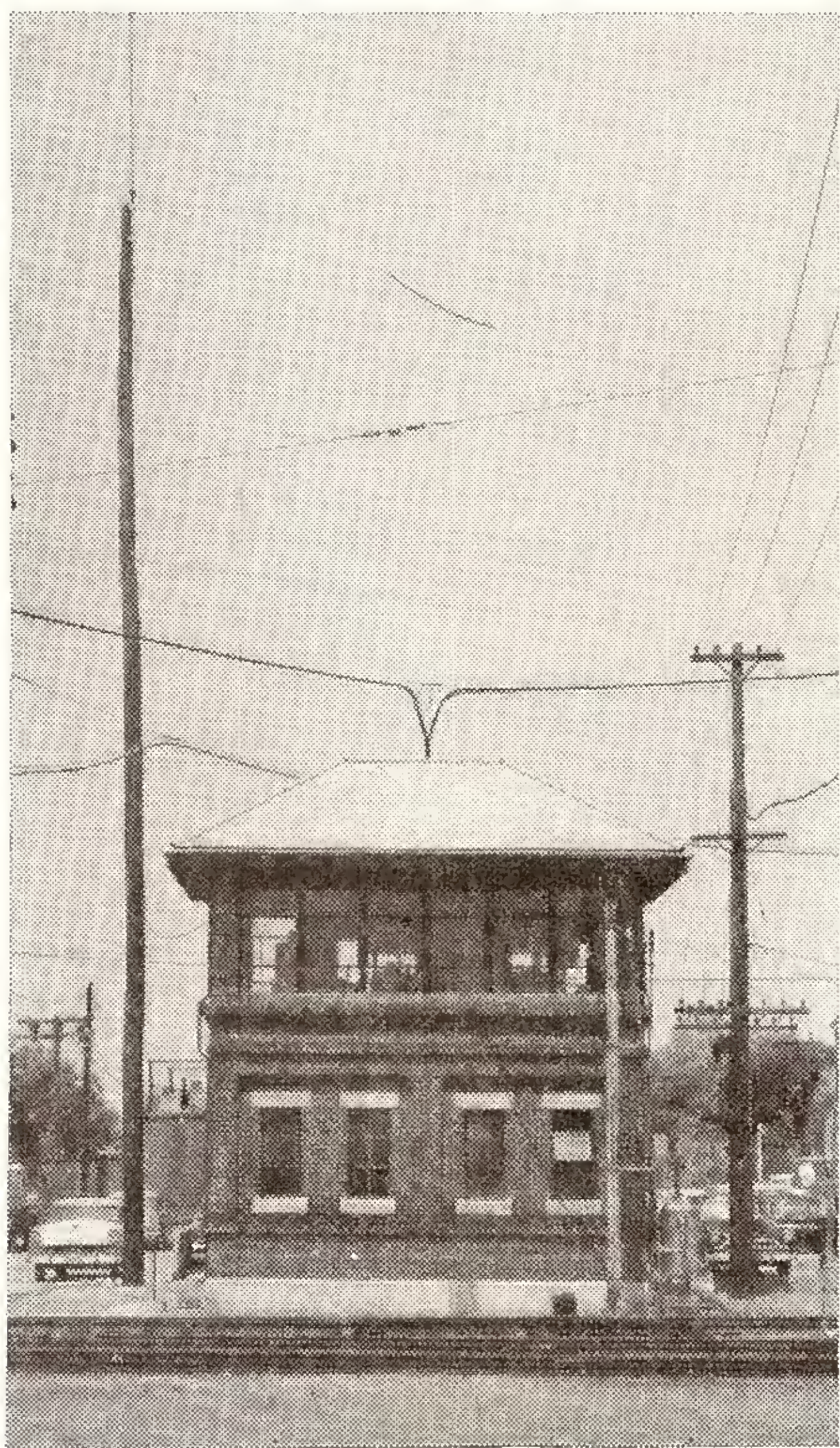
Ninety-foot antenna pole beside Ayer Tower provides widespread coverage for new wayside station radio system
