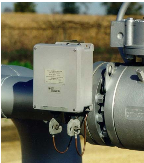
Figure 3-75: Solid State DC Decoupling Device
