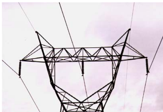
Figure 3-40: Typical Three-Phase AC Power Line (Horizontal Configuration with Two Shield Wires)
