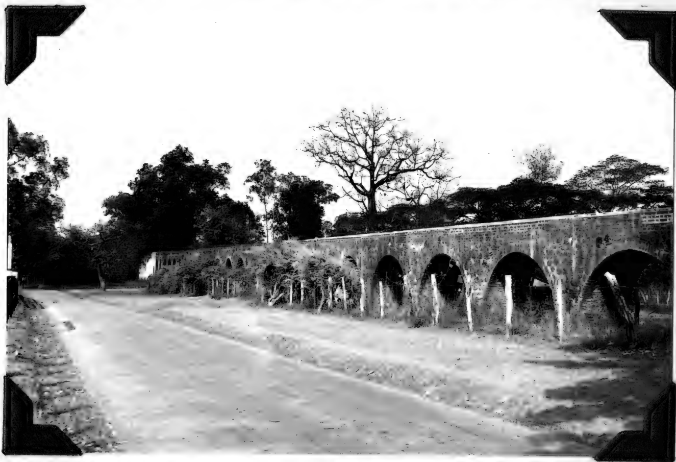
Old Spanish aqueduct still in use at Hope Gardens.
