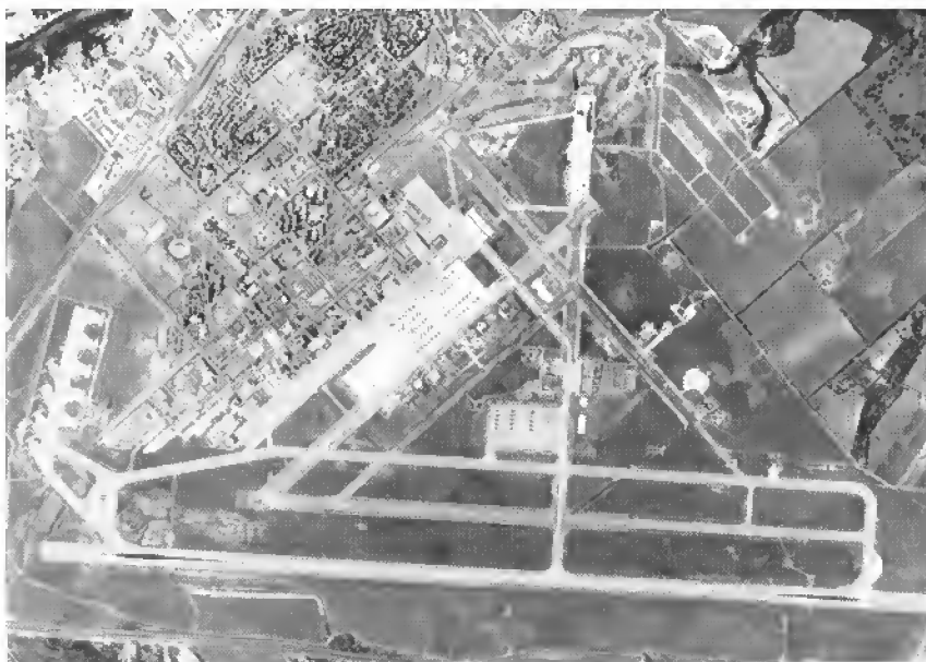
Bergstrom AFB, July 1984
