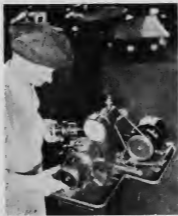
Grinding Cutters on 375-1 Cutter Grinder
