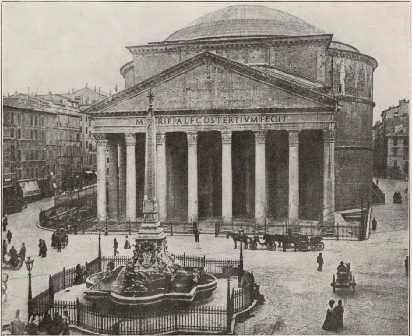
The Roman Pantheon—Concrete Dome nearly 2,000 years old—Rome, Italy
