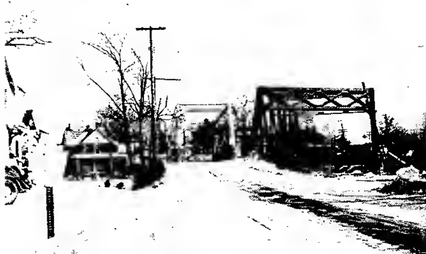
Traffic was maintained on the old bridge while the present bridge at the edge of town was being constructed.
