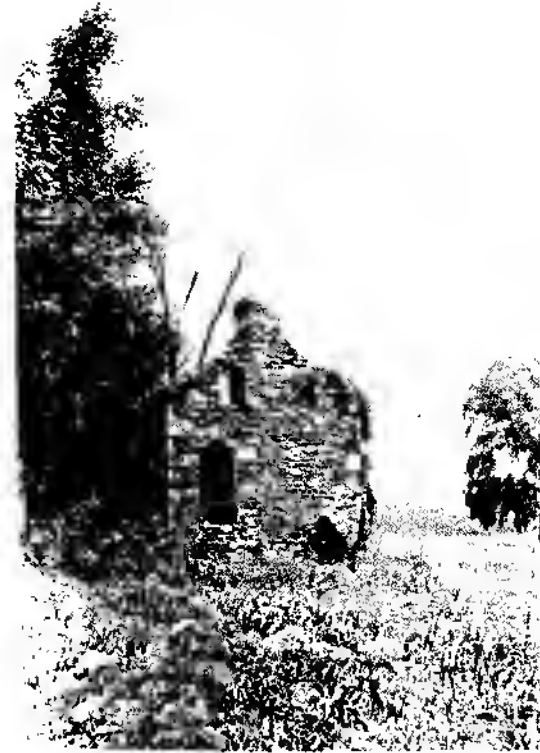
This house, built in 1800 and crumbling for the past eighty years, is still in evidence on the Bossert farm.
