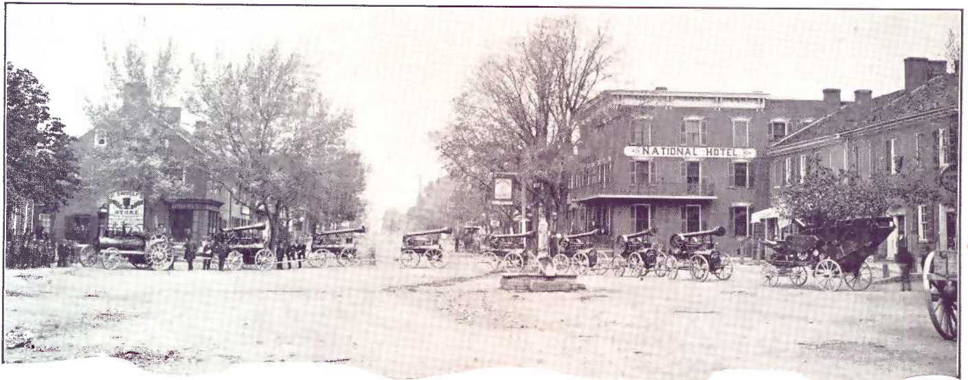
An early traction engine hauling seven portable engines and a thresher of the old "separator" type through Waynesboro's Center Square. Total load was 15 tons: the power of the engine amazed teamsters. Note the town pump, at which Gen. Robert E. Lee is said to have watered his horse in 1863; this photograph was made 20 years later.
