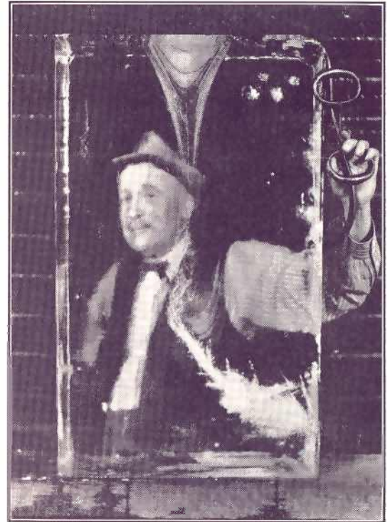
Ice made with the medium-pressure air system, using a tube in the corner of the can.
