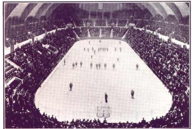
Approximately half the artificial ice skating rinks on the Continent, including this one at Hershey, Penna., have Frick equipment. We furnish rinks with or without cement floors.
