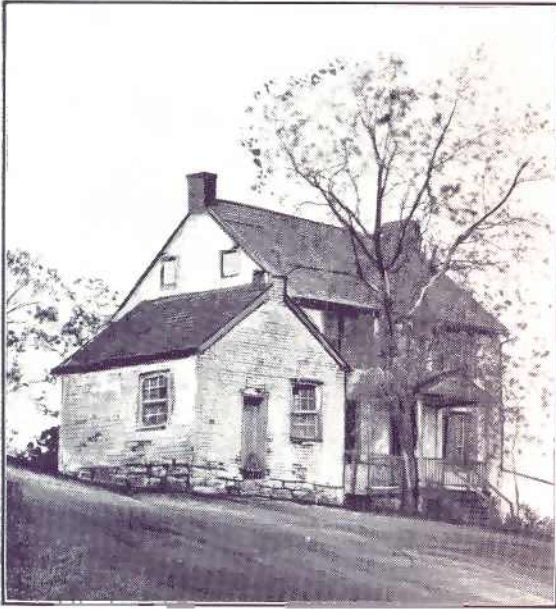
George Frick's shop and home near Ringgold, Md. His parents and a brother continued to live here after George moved to Waynesboro. The residence and shop still stand.
