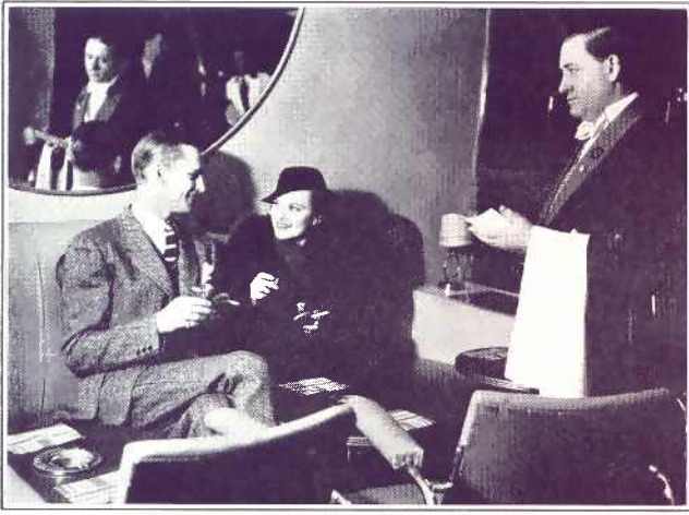
Jack Dempsey's Restaurant, opposite Madison Square Garden in New York City, was air conditioned with Frick equipment in 1935. Frick refrigeration was installed for food service and for cooling a display window.
