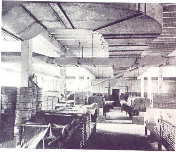
One of the first Frick air conditioning systems was installed in 1910 in this plant making caramel candy in Lancaster, Penna., where it served satisfactorily over 25 years.
