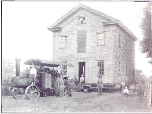
Moving a 30-ton house half a mile with a Frick traction engine. These machines crushed stone, built roads, pumped water, operated mills, and did many other kinds of belt and drawbar work.
