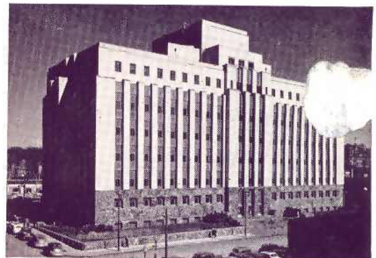
The "outstanding building of the decade" was that of the Bankers Life Co. at Des Moines. Costing $1,500,000, it included advanced methods of traffic control, space saving, communication, fire protection, and air conditioning. Three large Frick compressors, handling Freon-12, furnished 630 tons of refrigeration—and are of course still doing it.
