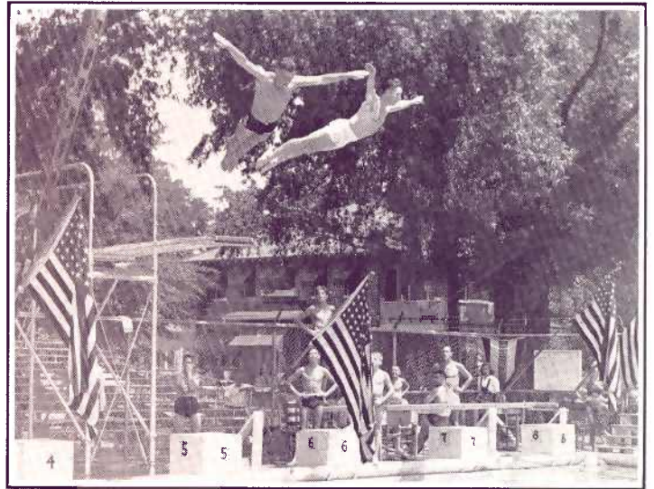
The water in the swimming pool at Tarboro, N. C., scene of many championship meets, is held at correct temperatures with a Frick ammonia system.
