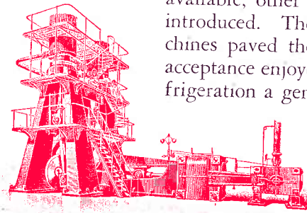
350-ton compressor shown in service above.
