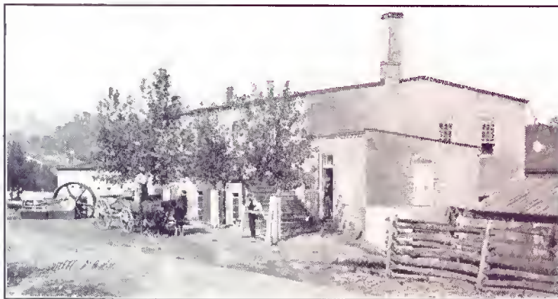
The "Brick Shops" were built across the street from the first Frick plant in Waynesboro, and were occupied from 1869 to 1881. They included a foundry, boiler shop, smith shop, forge shop, pattern dept., machine shop, etc.
