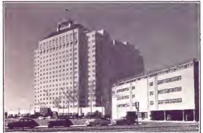
Frick equipment serves the $21,000,000 Shamrock at Houston, among other prominent hotels throughout the world.
