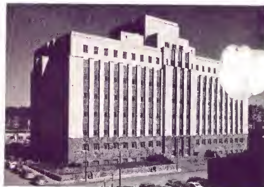
The "outstanding building of the decade" was that of the Bankers Life Co. at Des Moines. Costing $1,500,000, it included advanced methods of traffic control, space saving, communication, fire protection, and air conditioning. Three large Frick compressors, handling Freon-12, furnished 630 tons of refrigeration—and are of course still doing it.
