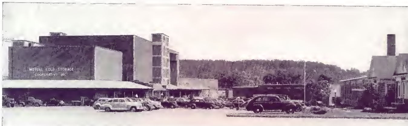
Six-story cold storage building, refrigerating machine room with ice-making system, and poultry packing plant near Broadway, Va. This big COMMUNITY REFRIGERATION CENTER, which includes a quick-freezing tunnel, lockers, fruit storages, etc., is typical of many throughout the country supplying similar varied services. Frick Company fostered the development of these CENTERS and is proud of their rapid growth and usefulness.
