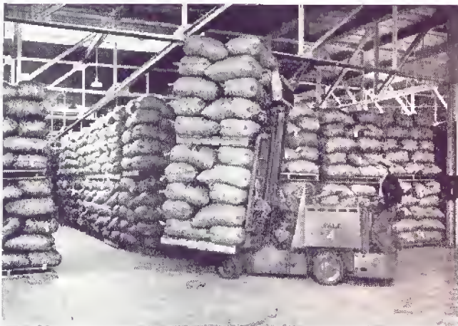
The great air conditioned storage of the California Walnut Growers' Assoc., at Vernon, measures 600 by 175 by 22 ft. high. The immense space is held between 36 and 40 deg. F. by two Frick 9 by 9 ammonia compressors, installed in 1936. A relative humidity of 65 per cent is maintained.
