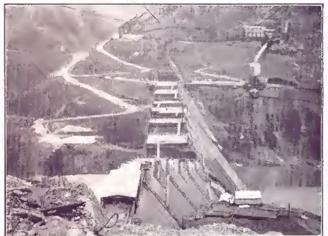
Frick engineering services, from layouts to test runs, are complete. Below is Detroit Dam, in Oregon, where the water, cement, sand, and even the rock used in making concrete are all pre-cooled to below 50 deg. F.
