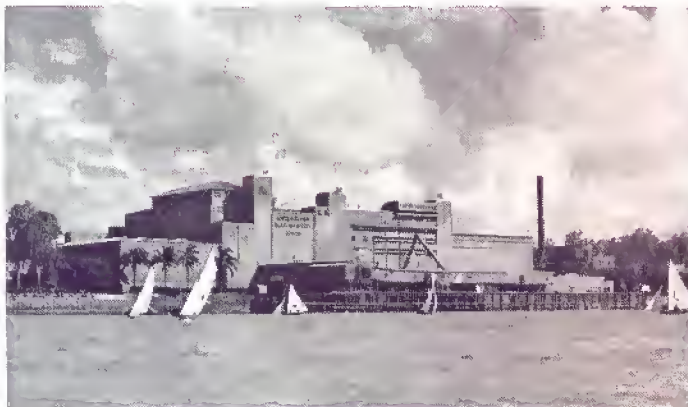
The Brisbane plant of the Queensland (Australia) Meat Industry Board, handling over 1,000,000 animals a year, increased its freezer output 26 per cent with three large booster compressors—typical of the important work being done overseas with Frick equipment.
