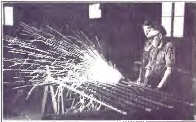
Left: Electric butt welding eliminated many screwed and flanged joints in cooling coils. End pressure, applied to the white-hot metal, thickens the walls at the joint, making the weld stronger than the pipe itself.
