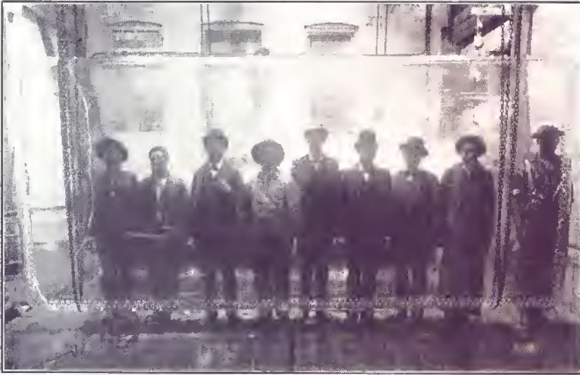
Sheet of clear ice made by the plate system. Single pieces measured up to 16 feet long and a foot thick; they might weigh 7½ tons. Two such sheets were frozen on opposite sides of a compartment of the tank. In the early days they were cut into blocks by steam-driven saws.
