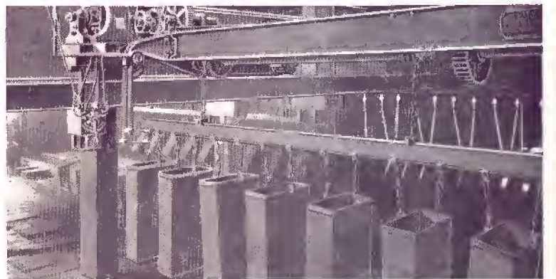
Probably the first group lift plant in America, installed at St. Louis in 1897. Thirteen cans were handled at a time; crane was electrically operated.
