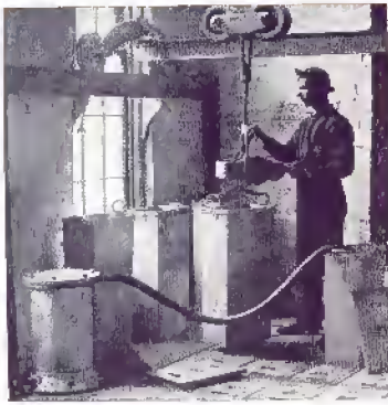
Showing methods of filling and harvesting cans in an ice plant of the 1880's.
