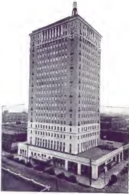
Seventeen tons of air conditioning for the Coffee Shops were included in the complete Frick refrigerating system installed in the Thomas Jefferson Hotel at Birmingham in 1929.
