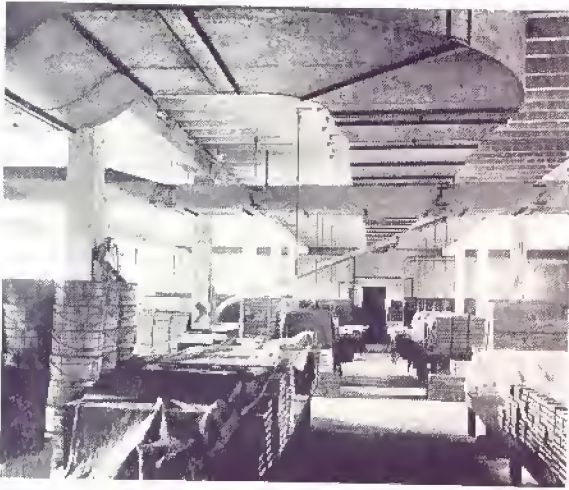
One of the first Frick air conditioning systems was installed in 1910 in this plant making caramel candy in Lancaster, Penna., where it served satisfactorily over 25 years.
