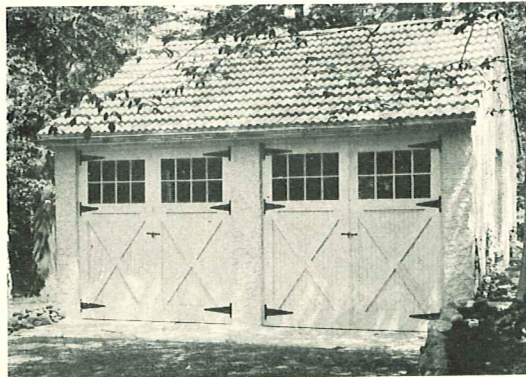
Walls of concrete masonry and portland cement stucco and roof of concrete tile give maximum fire protection to the garage
