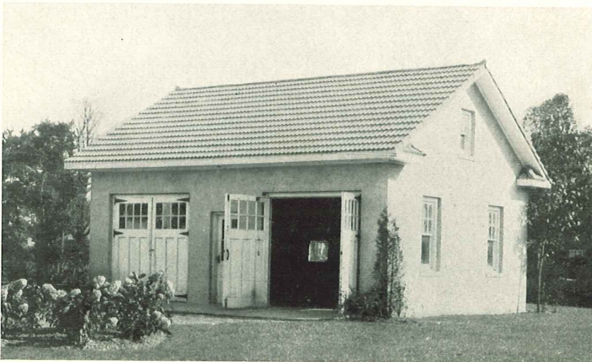
If not needed for car storage the extra space in a two-car garage serves as a good storeroom for garden tools. It also provides accommodations for visiting cars
