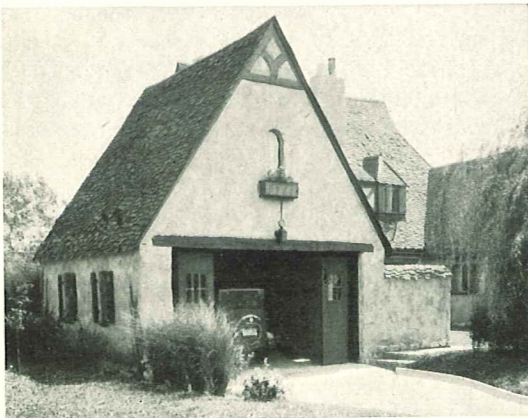
To obtain unity of appearance a predominating feature of the house design is often incorporated in the lines of the garage
