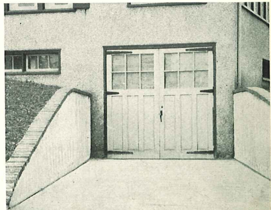
Where the lot slopes sharply to the street the garage is often planned and conveniently built as a part of the basement
