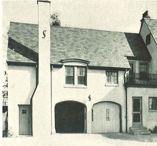
Above—When the garage is built as part of the house, the fire-safety afforded by concrete masonry is not only an advantage but a necessity
