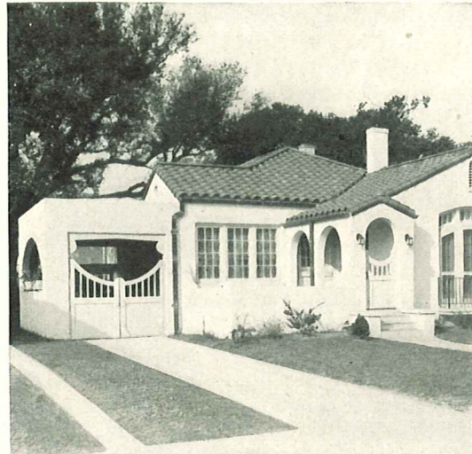
Above—When the garage is built as part of the house, the fire-safety afforded by concrete masonry is not only an advantage but a necessity
