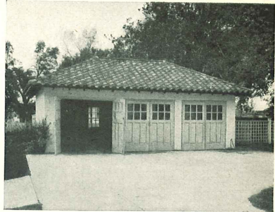
The cost per car of building a garage for two or more cars is relatively less than for a one-car garage
