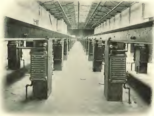
Used in car barn repair pits, in conjunction with AMERICAN Colonial Radiators for melting snow and ice from running gears of street cars.
