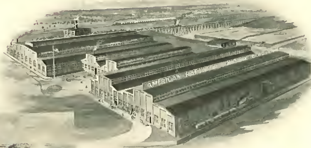
Bond Plant, at Buffalo, N. Y. (Run by Niagara Falls Power)
