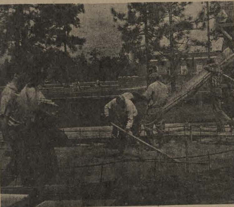
Construction progresses on Armstrong's mid-campus fountain. photo by Tom Lovett
