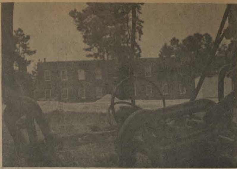
Construction begins on the new classroom building.
