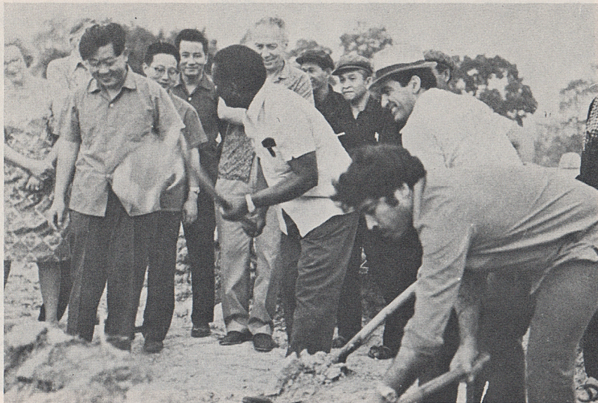
AMBASSADORS AND DIPLOMATS FROM FRIENDLY COUNTRIES PARTICIPATE IN THE CONSTRUCTION OF EMBANKMENTS OF RICE FIELDS AND IRRIGATION CANALS. (GEORGE HILDEBRAND)
