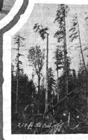
Topping a Spar Tree
