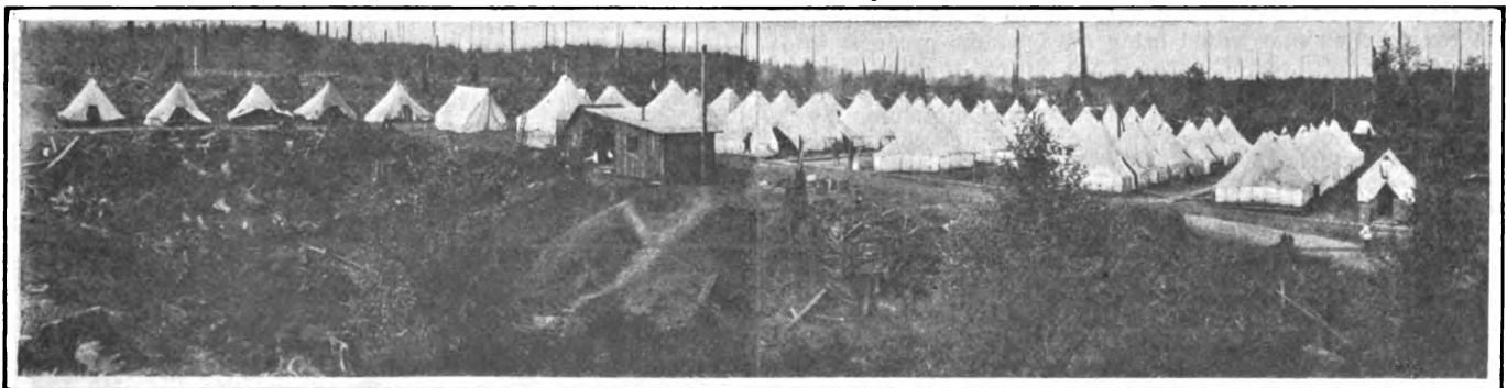
Where Some of the Construction Crew Camped During Building of Olympic Peninsula Railroad
