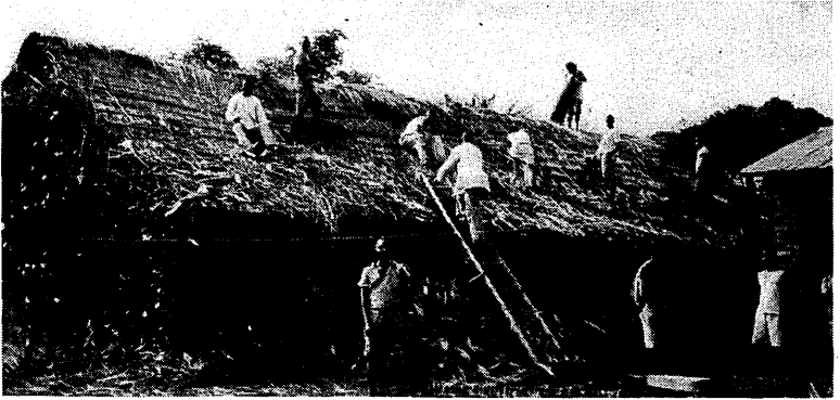
Replacing the Roof on a Missionary Home, Congo.
