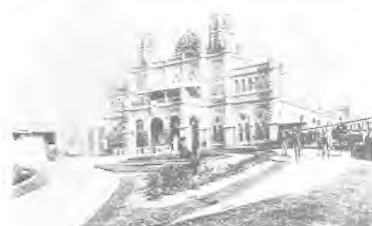
The Exhibition building, probably taken at the time of the 1897 International Exhibition, the year of Queen Victoria's Jubilee—celebrated in the banner hanging over the front entrance in this photograph.
