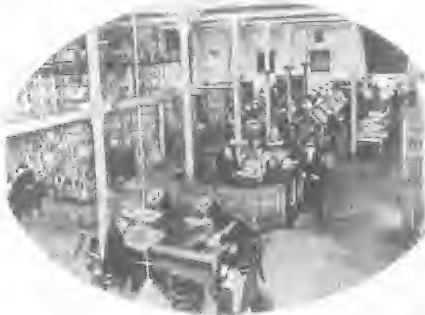
The ground floor of the State Library in 1930. Apart from the mezzanine floor which was added after the museum moved out 30 years before, it is much as it was when it was the museum. The internal stairs to the basement can be seen beneath the mezzanine—behind the reception desk; the front entrance is to the right of the photograph and the stairs to the first floor are in the upper right corner (photograph by courtesy Oxley Library).
