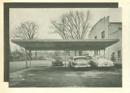
Built in standard sections, 30 or 36 feet wide by 18 or 20 feet long, which can be added to at any time.
