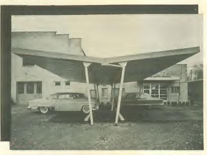
Requires simple foundation due to balanced design. May be used with center walkway, or arranged for bumper-to-bumper parking.
