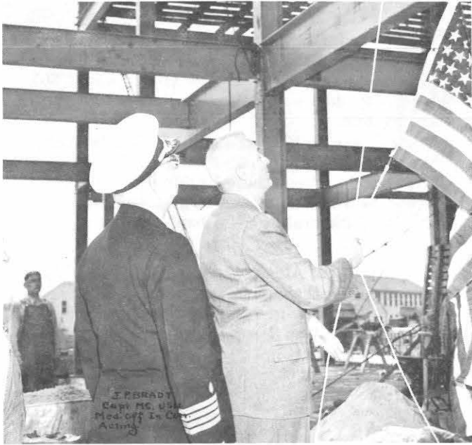
4-22-49: USNH St. Albans, N. Y. Topping of Steel Ceremony.
