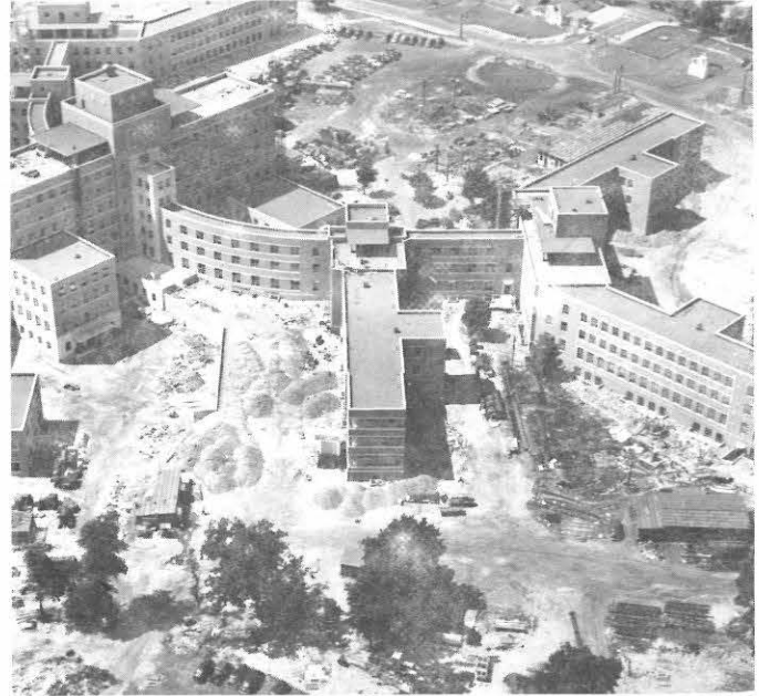
11-18-50: USNH St. Albans, New Construction Looking Southeast.
