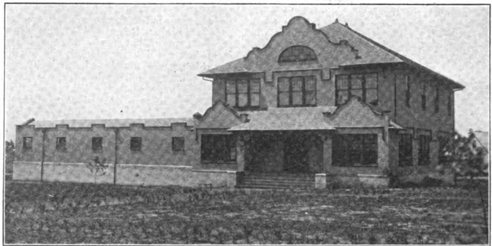
OPERATIVES' CLUB HOUSE
