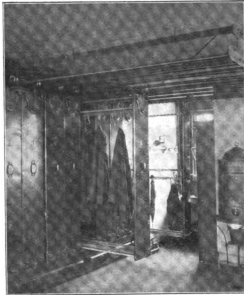
CLOTHES DRIERS, HEATED BY STEAM, BOSTON.
