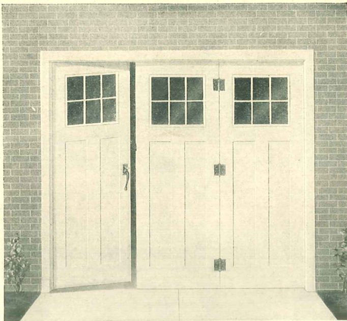
The appearance of garage from outside is enhanced by absence of any structural iron-work. Note how the one door opens without disturbing the others.
