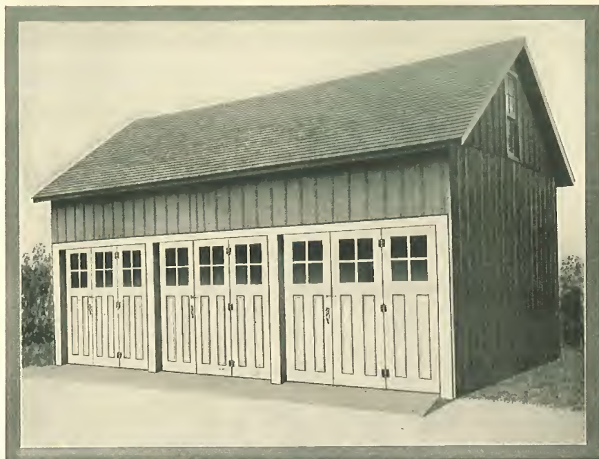
A practical method of remodeling an unused barn into a three-stall garage. An inexpensive method of converting an unprofitable building into a profit-producer. No skilled labor required. (Equipment, pages 18 to 21.)
