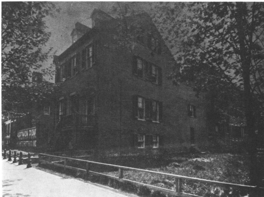
Fig. 1. —Southwest corner of 18th and K Streets, N.W., Washington, D.C. This building may have housed the Naval Dispensary circa 1880. We are unable to document this however.
