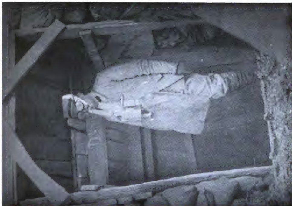
FRENCH SAPPER WITH RESPIRATION APPARATUS ABOUT TO ENTER A GALLERY AFTER A MINE EXPLOSION
