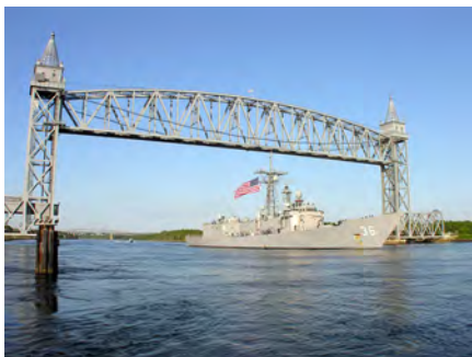
Underwood passing under the Cape Cod Canal railroad bridge, June 2006
