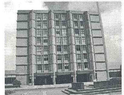
Letterman Army Medical Center, to be demolished.
