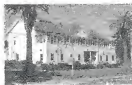
Buildings 36 (above) and 50, the Officers' Club (below), are among the historic buildings on the Main Post.
