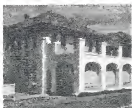
Part of the rehabilitated historic Letterman Hospital, now the Thoreau Center for Sustainability.
