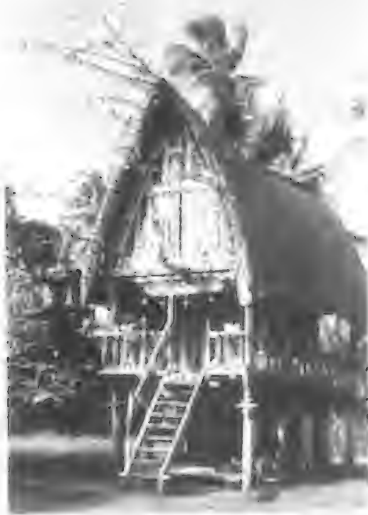
FIGURE 3. Chief's house ( tipua ). Note gable boards ( kaivaipahu ) and tasaha with pendant mana shells, the kaduguwai project from the peak of the gables (Photo: R. Lawton, 1972).
