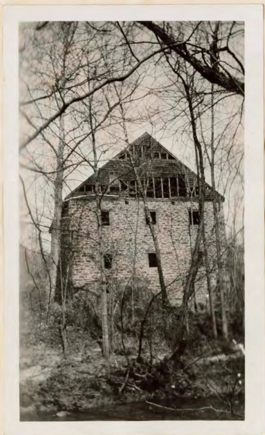
Figure #2 South View of Mill
