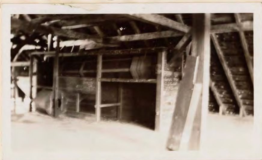
Figure #6 Third Floor of Mill
