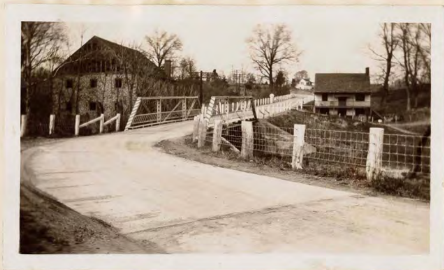
Figure #1 South View of Mill & Mill House
