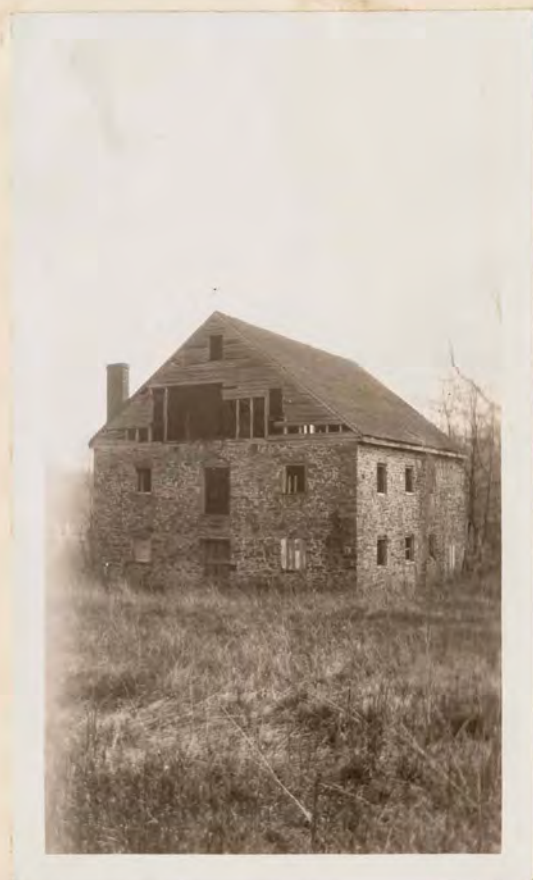
Figure #3 North View of Mill
